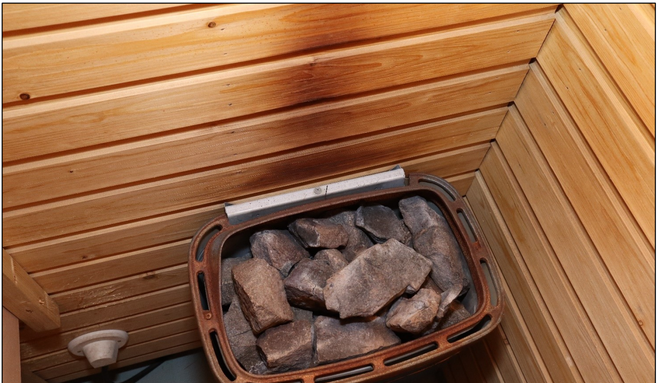
Figure 15. The sauna heater in another apartment in the building where the accident happened. The panel wall above the heater has darkened significantly. Some of the topmost stones on the heater were quite large. (Photo: Safety Investigation Authority, Finland)
