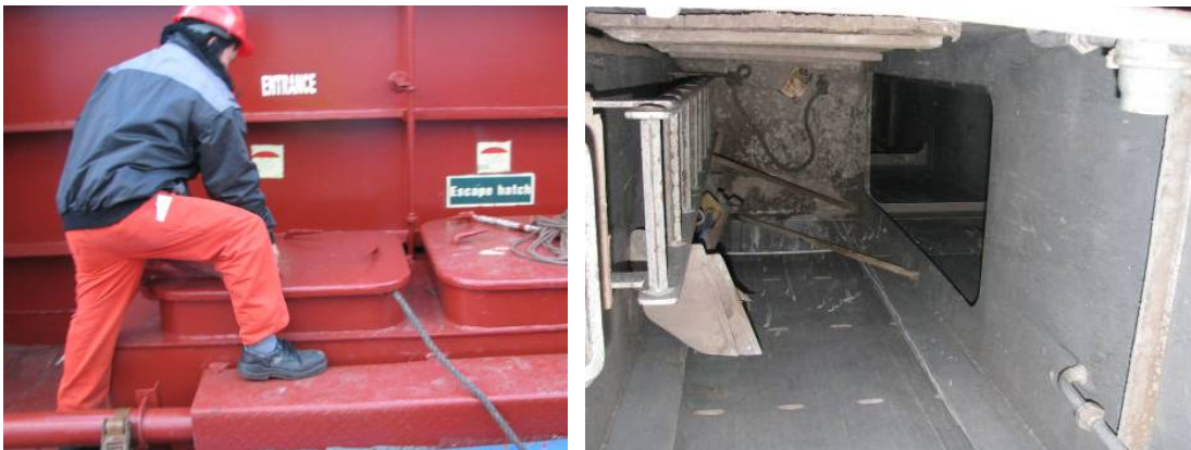
Figure 4. The manhole of the cargo hold to the left. The ladder leading to the hold and the landing, photo taken towards the bow.
