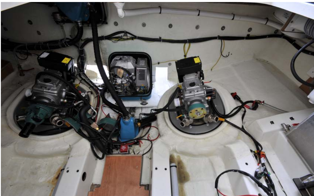
Figure 3. The rear part of the bottom frames has been replaced by a Volvo Penta mount ring and the stringers supporting it. The picture was taken after the engines were demounted and the engine compartment was cleaned.
