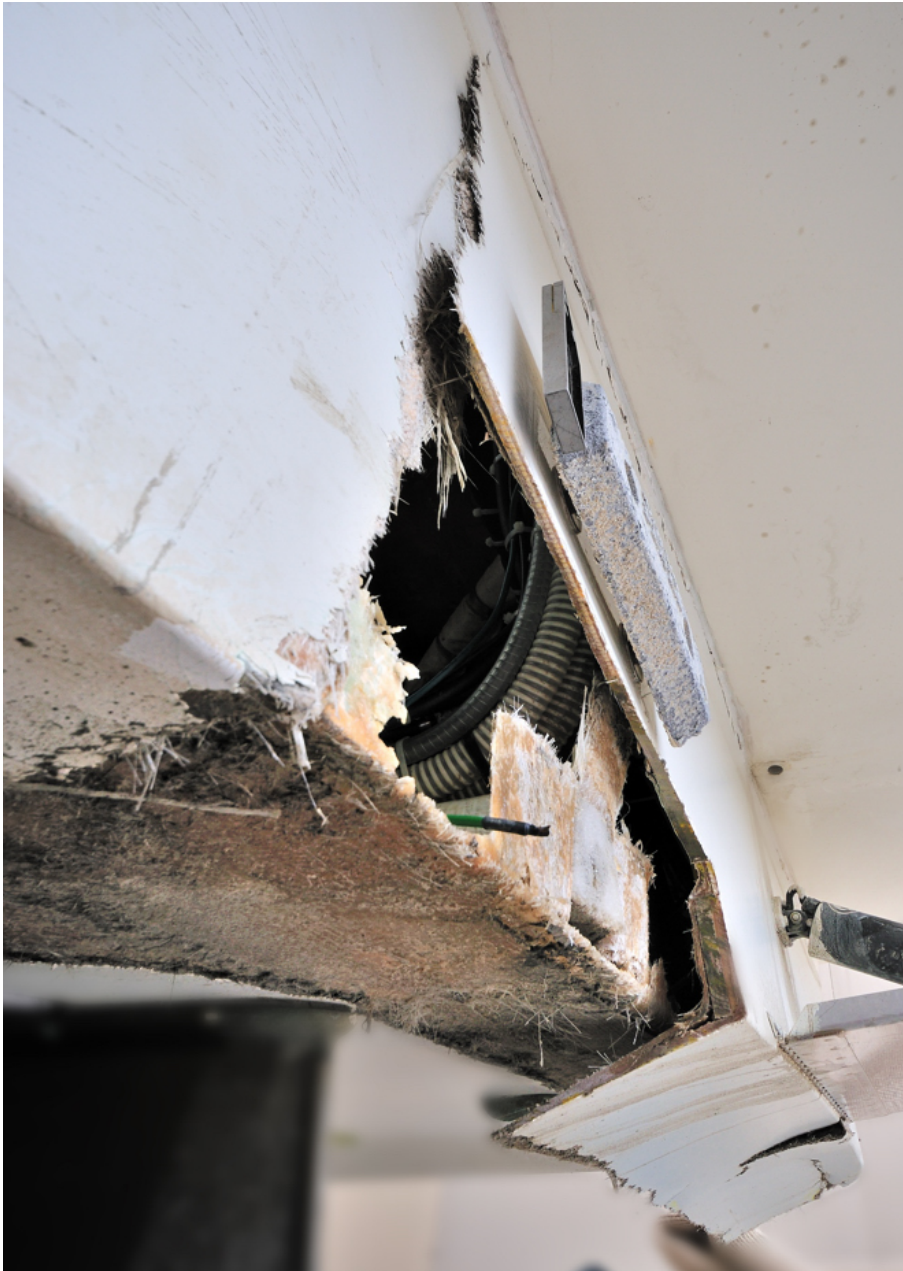
Figure 30. In the picture taken after the test sample had been cut it can be clearly seen how the transom and the bottom have torn loose from each other. Reinforcement layers have not been lapped in turns but the transom has been completed first and the bottom of the boat has been laminated on it (in a mould). The parts have come loose from each other along the joint between them. The bracket attached in a careless manner between the transom and the IPS mount ring can also be seen in the picture.
