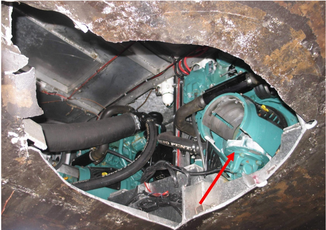
Figure 1. The hole cut in the bottom of IDA 1 after the drive unit had been dismounted. The arrow points to the broken shaft coupling.
