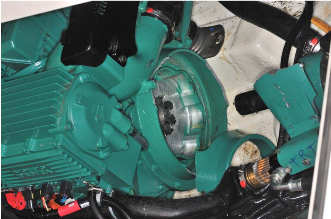
Figure 18. The broken flexible coupler and the metal casing broken by the shaft.
