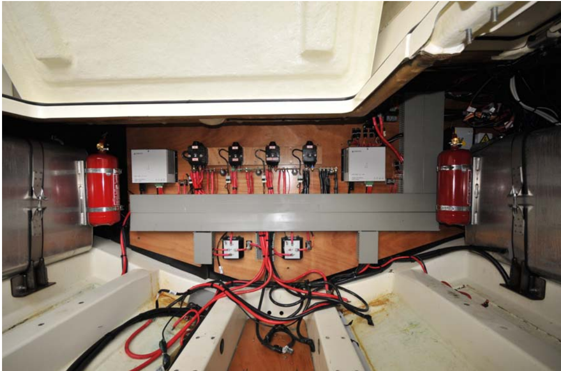
Figure 4. The structure of the bottom at the engine compartment.
