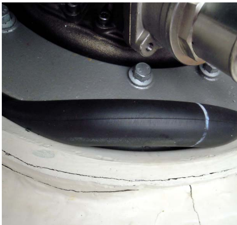
Figure 23. The O-ring between the drive unit and the glassfibre mount collar had slipped out from its groove thus generating an extra point of leakage. Note also that the laminate had broken at the mount collar.
