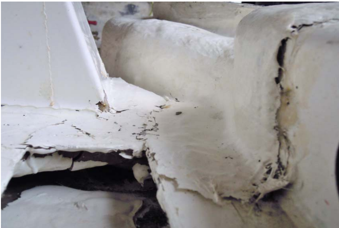
Figure 28. The stringers of the bottom and jointing them to the mount ring. According to the investigators' view, all the gaps visible in the picture have not been caused by the accident but the parts have been loose from each other already before the accident. This is indicated e.g. by the topcoat partly flowing down under the joint surfaces. The strength of the structure is questionable considering the fact that in an IPS drive unit the thrust moves to the hull by the transmission of this structure.
