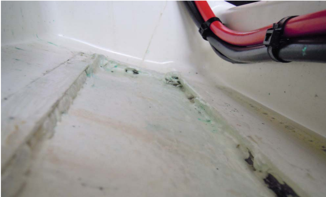
Figure 27. Bottom stringers have been jointed to the hull with glue mass. The fitting of the parts has not been accurate.
