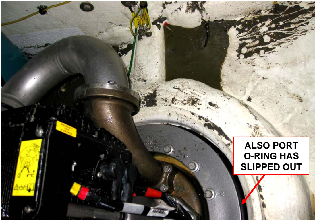
Figure 24. The O-ring of the port drive unit had also slipped out even though the impact on this drive unit was weaker.
