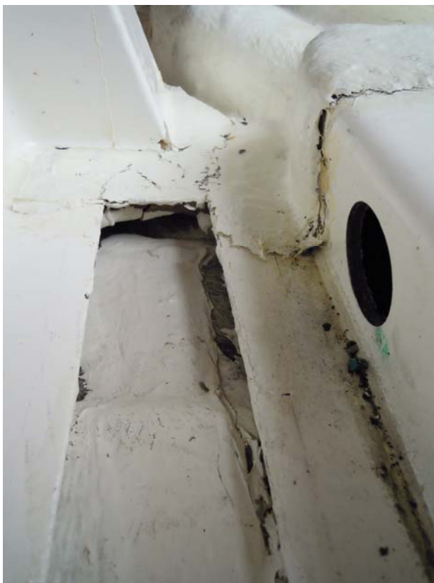
Figure 5. The way the bottom frames are jointed to the hull. The stringers were not completely jointed to the bottom. The fitting had been done by using glue filler.
