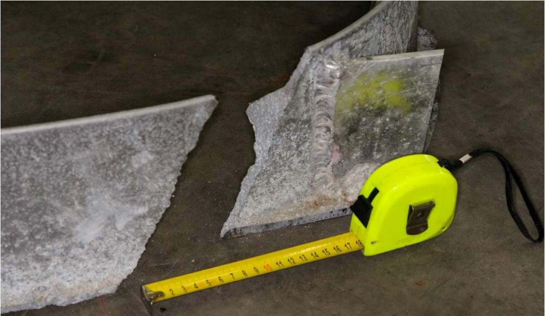
Figure 9. Breakage point of the aluminium collar.
