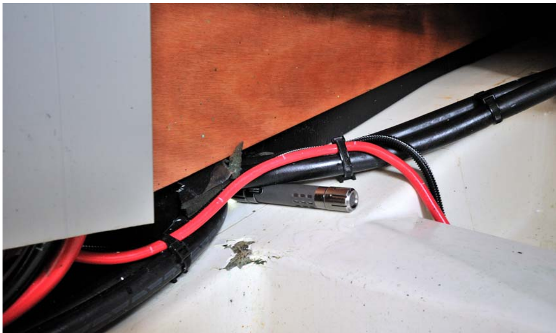
Figure 33. The gap between the plywood bulkhead and the glassfibre structure was filled with Styrofoam. It serves as the lead-through point for hoses and cables. By the way of example, also the hand torch of the investigator has been pushed under the bulkhead in the picture.
