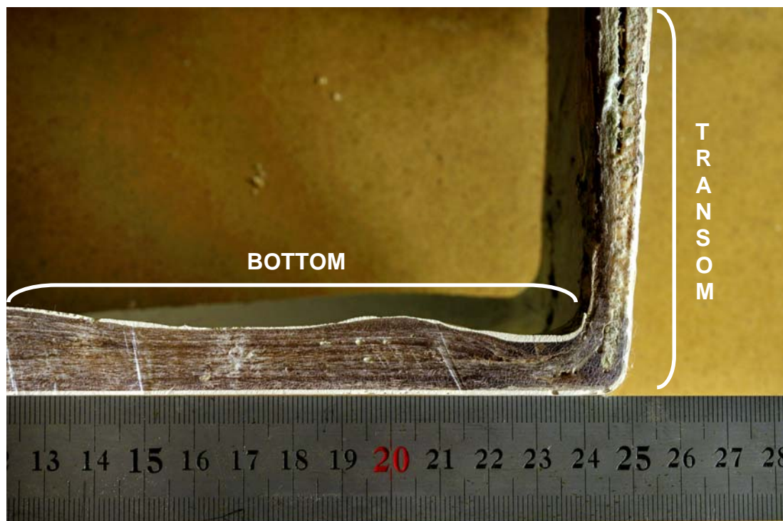
Figure 14. The picture shows a test sample cut from the hull of the boat, from the area where the bottom and transom come together. The test sample was cut off from the port side of the hull, which had remained intact, i.e. where the laminate had not torn. The thickness of the transom is at its lowest approx. 8 mm as shown in the figure. Approx. two 1.5-mm layers of this are glassfibre laminate. Between the laminates there is filling material which appears to be microbead mass and which makes the texture sandwich structure.
