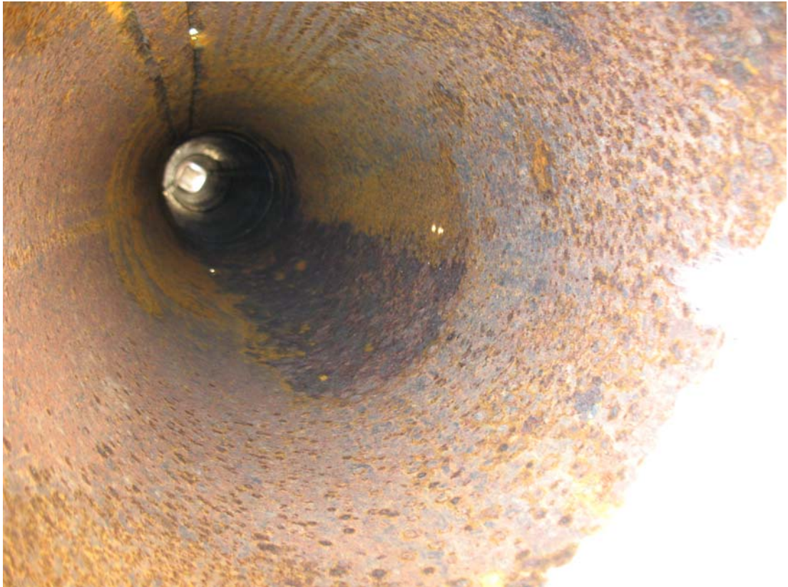
Figure 10. Corrosion inside a mast. (FMA)
