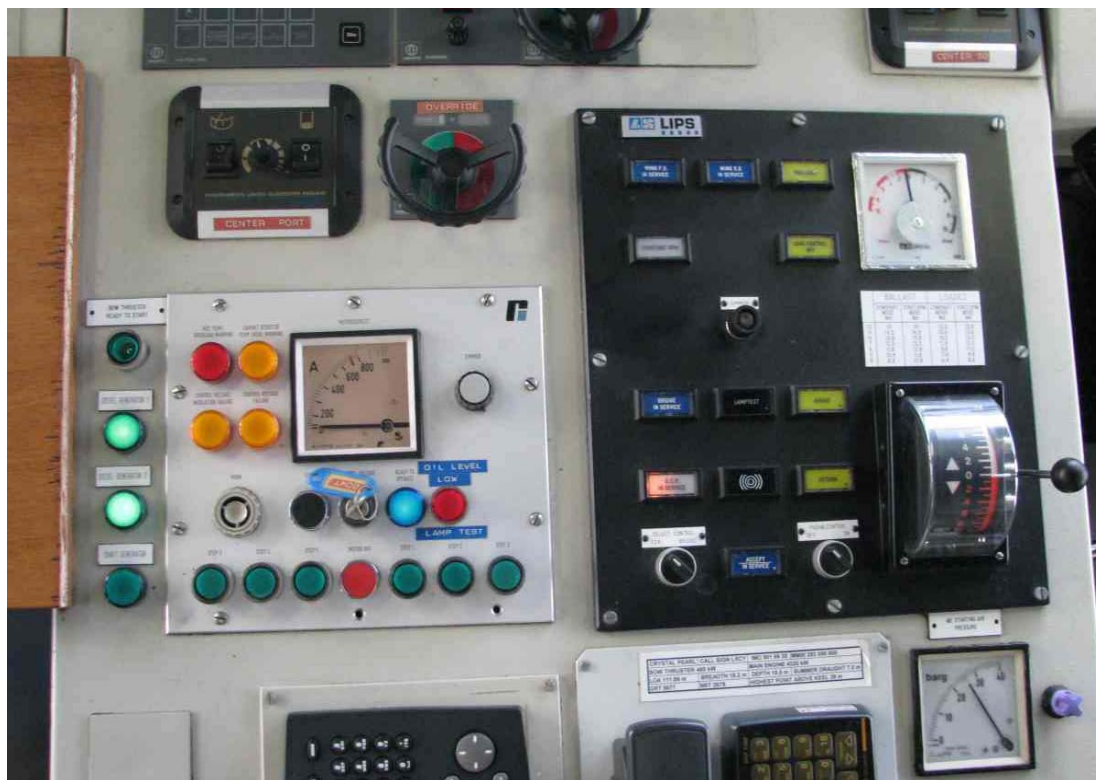
Picture 7. The control panel for the bow thruster on the left, the controls for the propeller pitch and RPM on the right.
