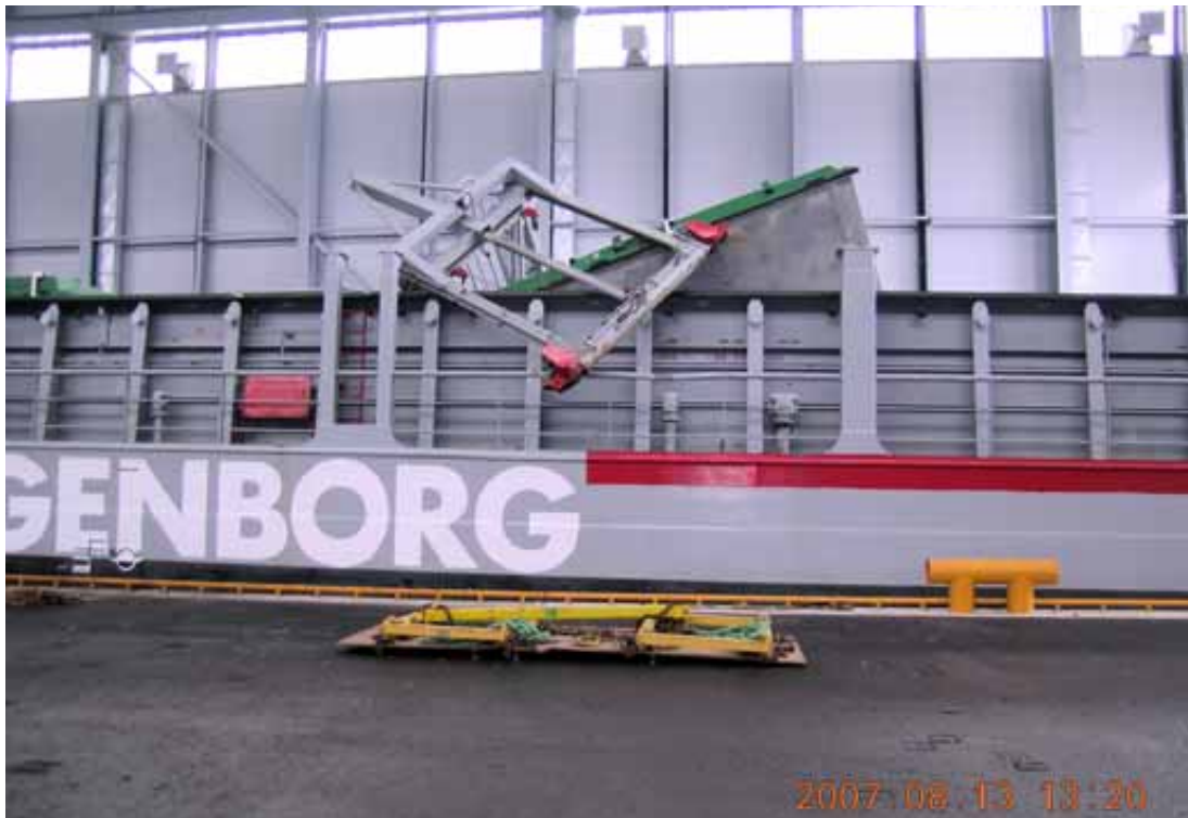
Figure 3. M/S GRACHTBORG's collapsed hatch crane.
