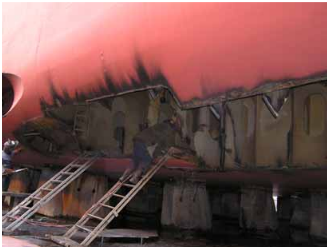
Figure 13. Part of the damaged section cut off portside of the stern of the vessel.
