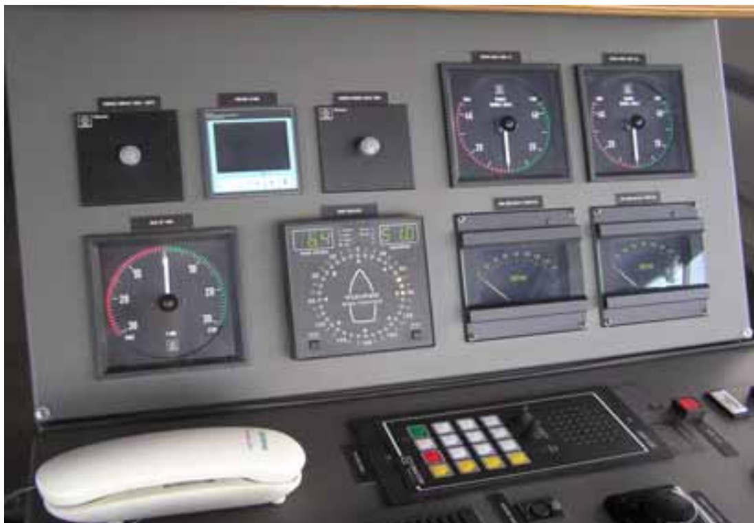
Figure 6. The indicator panel on the wing. The indicators from the top left: console light dimmers, mooring alarm, dimmer of rudder angle indicators and rudder angle indicator. Bottom row left to right: angular velocity indicator, wind gauge and tachometres of main propellers.
