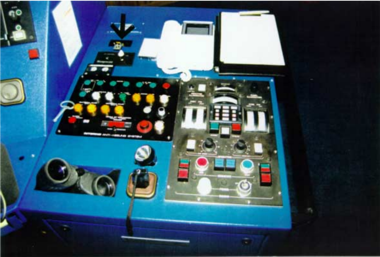
The right-hand side of the navigation desk. The arrow indicates the location of the BY-PASS switch.
