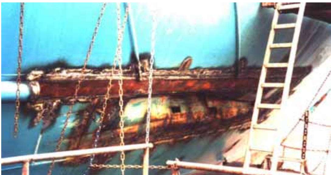
Figure 25. The damage on the side plating above waterline in bow, this is damage nr. 3 in figure 21.
