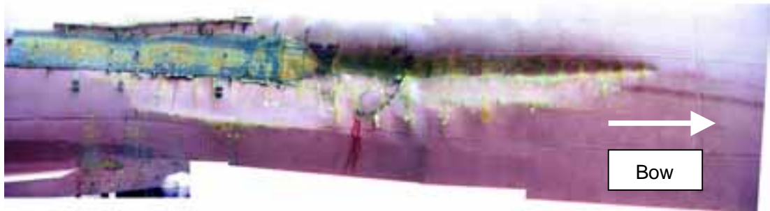
Figure 22. The damage on the side plating below waterline, damage no. 1 in figure 21. The cut is very sharp and the bow is to right. The hole is still temporarily repaired for the voyage from Turku to Germany. (Note that this picture is a composition and the perspective is not correct.)
