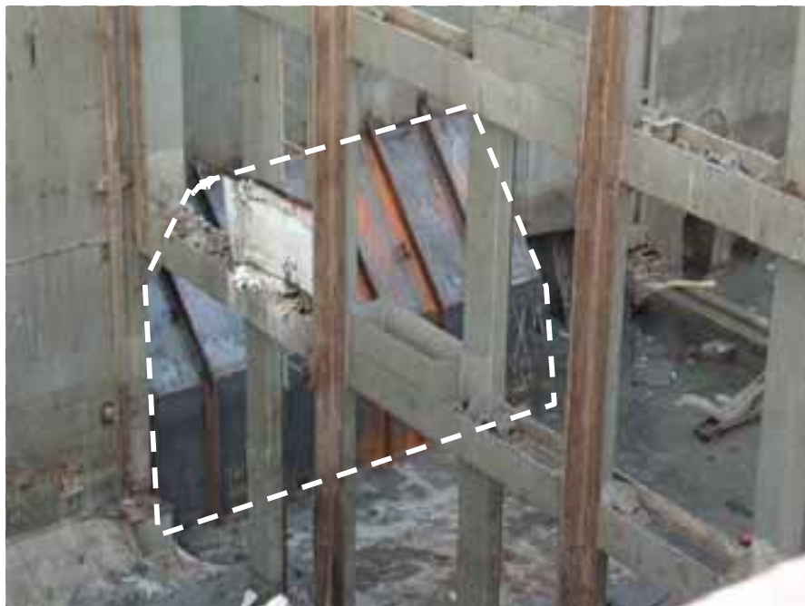
Figure 23. The temporarily repaired damage in hold no. 1.
