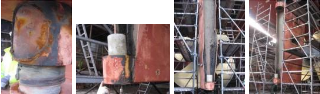
Figures 9, 10, 11 and 12. Damages to the rudder (photographed at the repair yard). (Photos: DNV GL)
