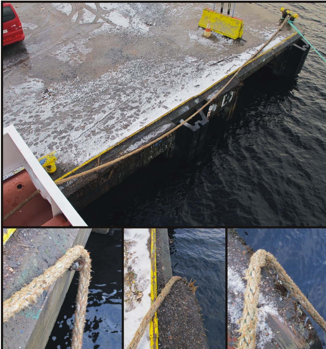
Figure 9. There were several points on the edge of the quay where the line could get stuck. Photo taken on 27.11.2013. (photos: the police)
