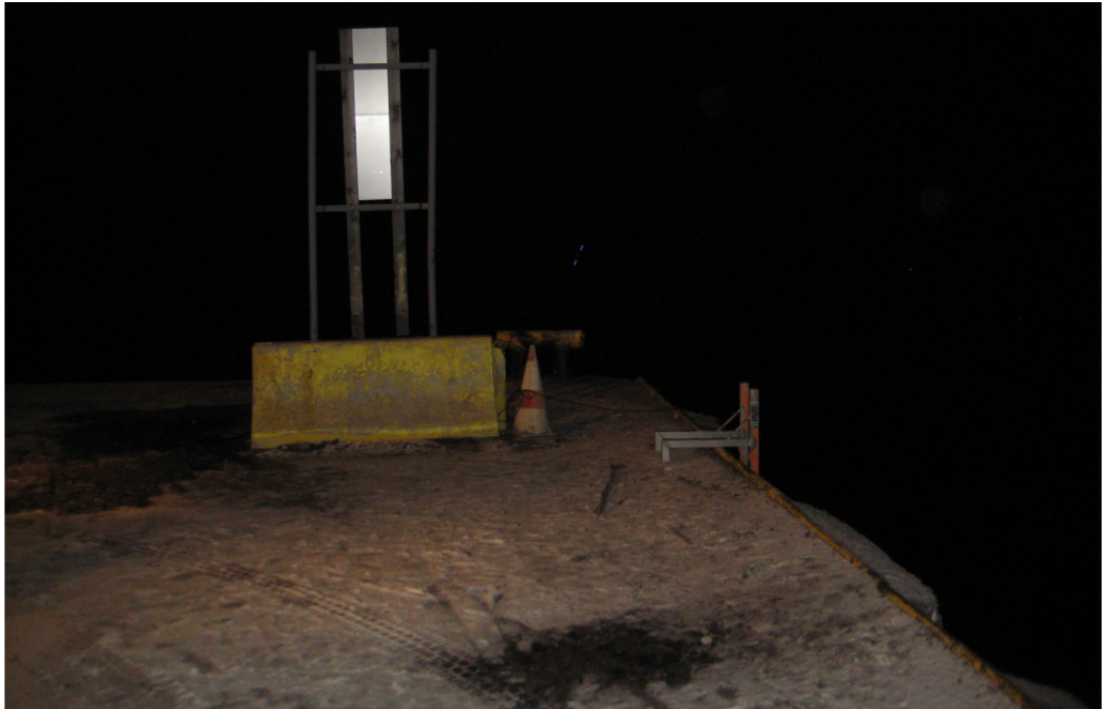
Figure 5. Photo of the scene of the accident 26.11.2013. The passageway on the edge of the quay was fairly narrow because of the concrete base of the information board and the attention cones stacked next to it. The ladder seen at the edge of the quay was brought there during the rescue operations. (photo: Stora Enso mill fire brigade)
