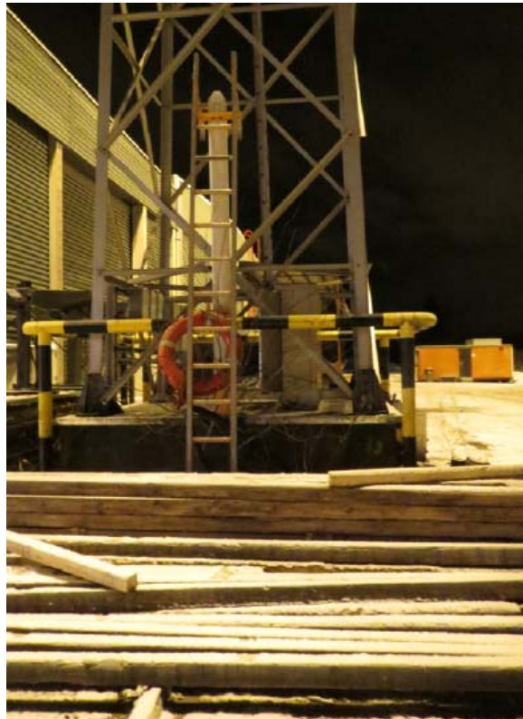
Figure 12. The ladder and lifebuoy near to the accident scene, photo taken on the evening of the accident 26.11.2013. The Government Decree on the Occupational Safety in Loading and Unloading of Ships requires that there must also be a round-tipped boat hook available. (photo: Stora Enso mill fire brigade)
