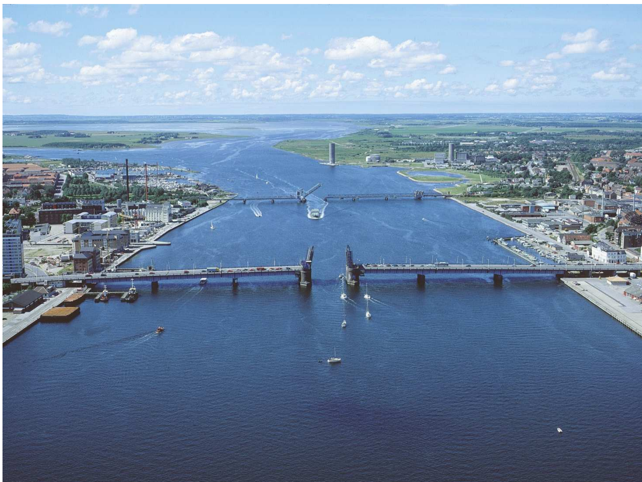
Figure 6: The Limfjord Bridge and the Railway Bridge viewed from the east with open bascules Source: National Survey and Cadastre
