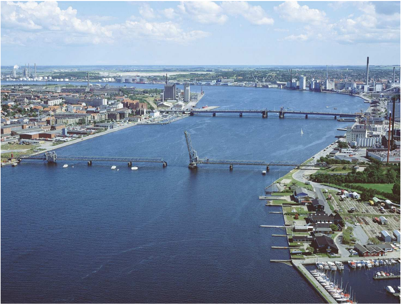
Figure 4: The Railway Bridge viewed from the west with open bascule, the Limfjord Bridge further away with closed bascule Source: National Survey and Cadastre
