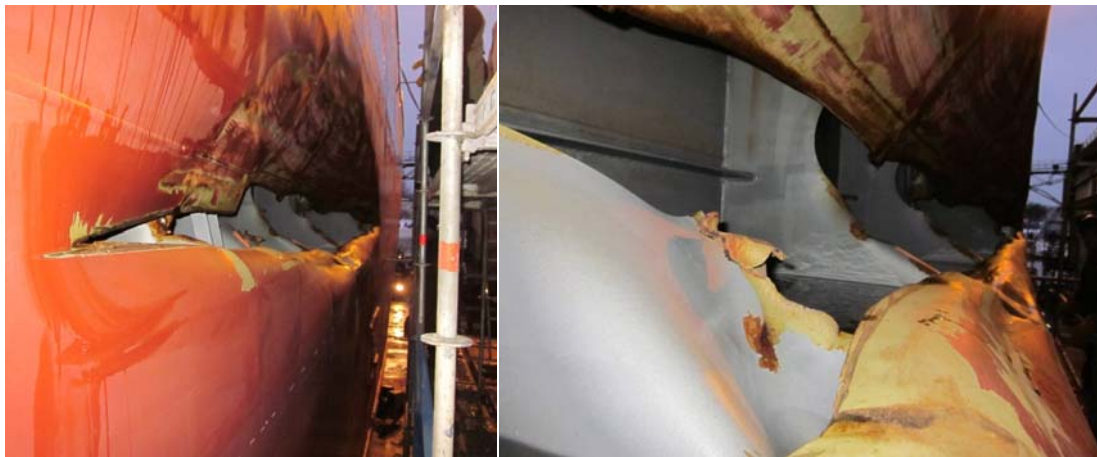
Figure 10. Damages on the port side.
