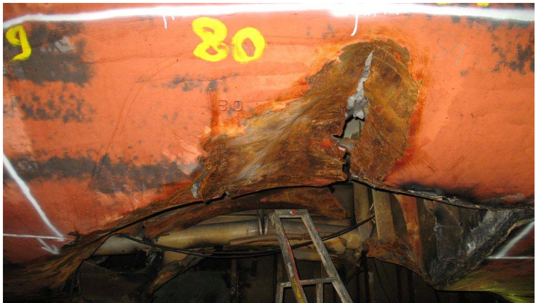
Figure 8. Damages to the vessel; tear in the starboard-side ballast tank.
