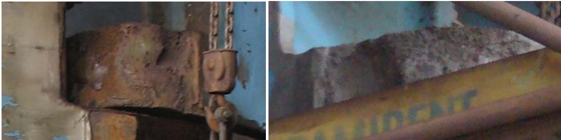
Figure 13. Cavitation corrosion in the rudder horn. BB to the left (photo taken on 3 December 2009), SB to the right (photo taken by the Finnish Transport Safety Agency on 4 December 2009), both on the side of midships.
