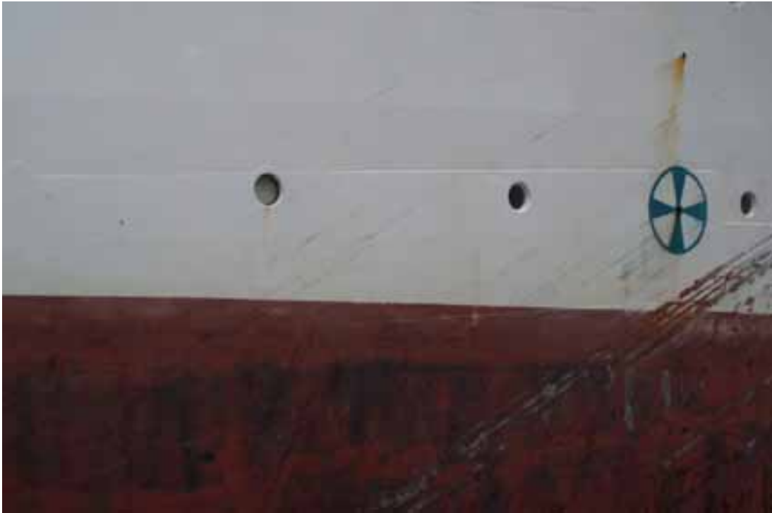
Figure 7. Broken valve on the starboard side of the vessel.
