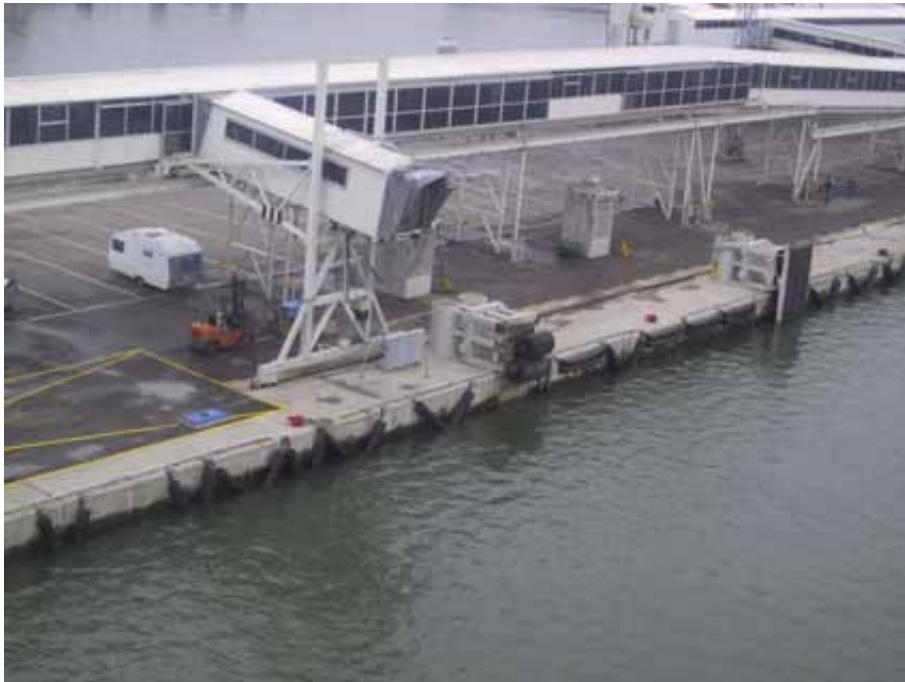
Figure 22. In the foreground the passenger gangway of the quay and the fender which were damaged by the NORDLANDIA's collision. In the figure the damaged fender located to the left has been repaired temporarily, and the intact fender can be seen to the right.
