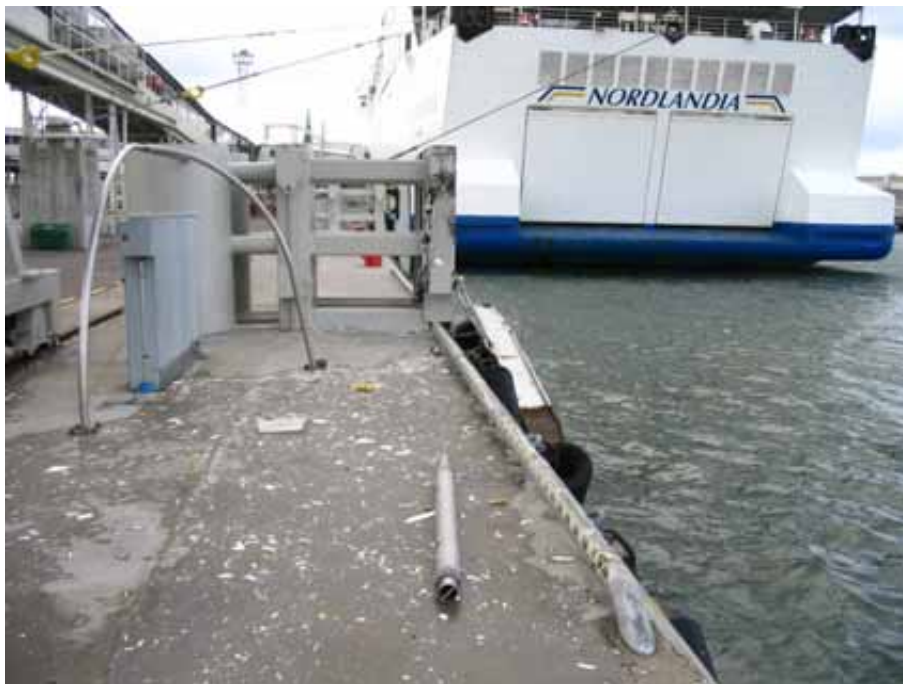
Figure 21. The damaged quay fender.
