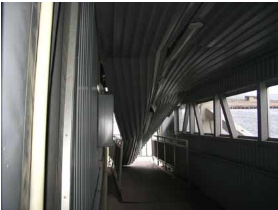
Figure 23. Damages to the passenger gangway.
