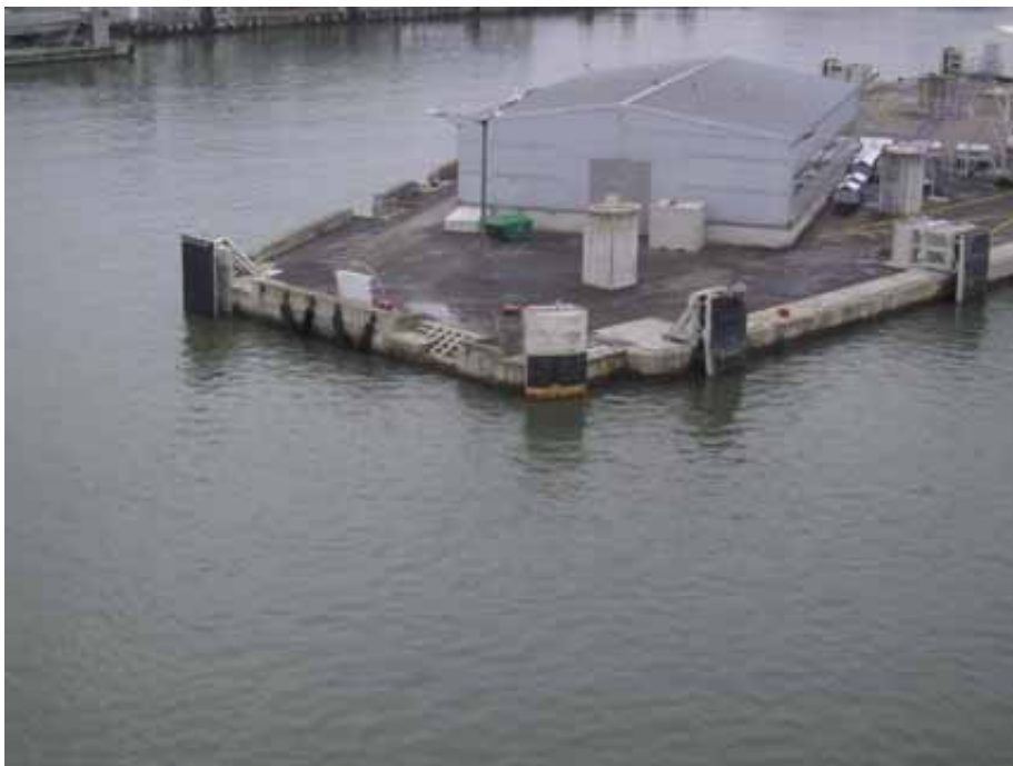
Figure A4b. There is a fender at the corner of the quay, and it can be used as support when the vessel is turned parallel with the quay.
