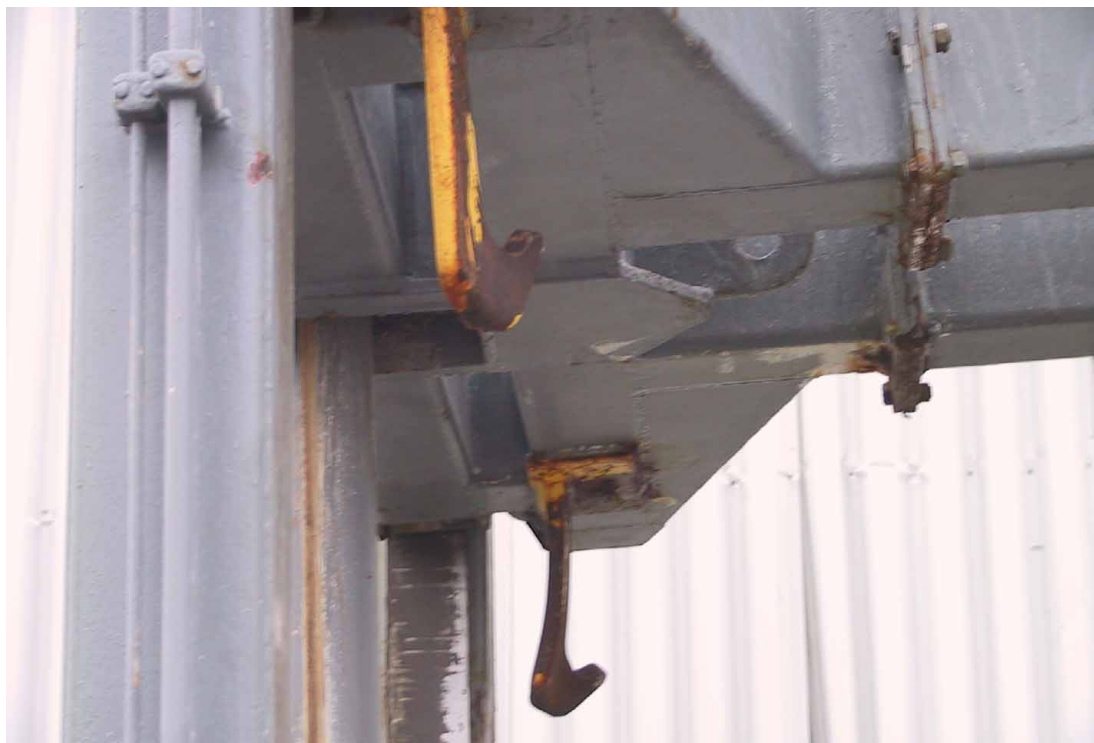
Figure 6. Twisted lifting hooks.
