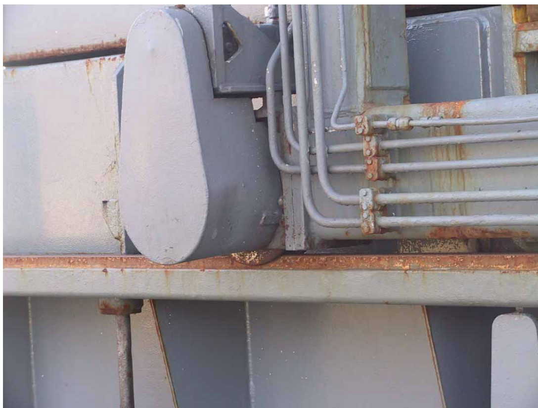
Figure 11. The rail wheel of the crane in a sister vessel.
