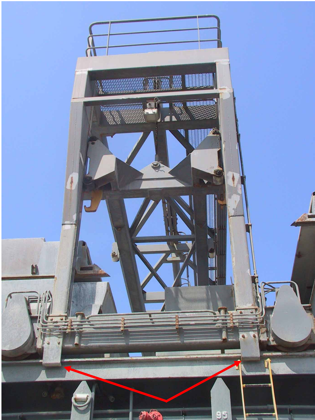
Figure 10. Crane equipped with safety catches. Red arrows point the safety catches.
