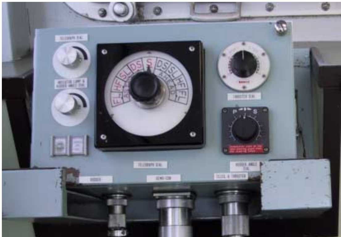
Figure 5. Controls on the starboard wing of the bridge.
