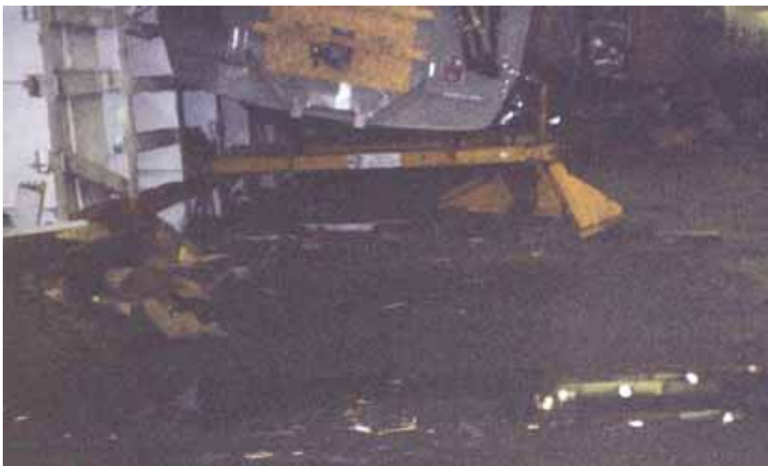
Figure 17. Railway carriage on the main deck and collapsed trestles.
