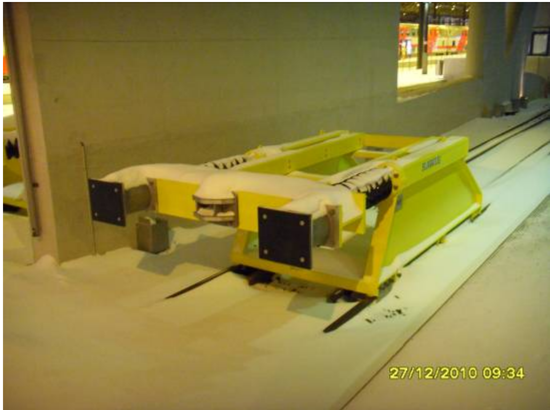
Figure 19. New rail barrier on track 13.
