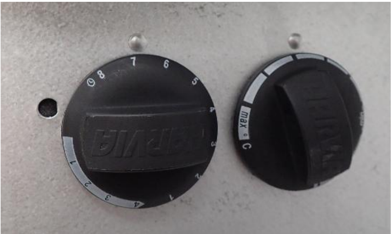
Kuva 5. Control knobs on a new sauna stove of the same make. The control knobs were in reverse order in the sauna stove of the flat where the accident occurred. The small hole on the left hand side of the photo is the reset button for the overheating protection. (Photo: SIA)
