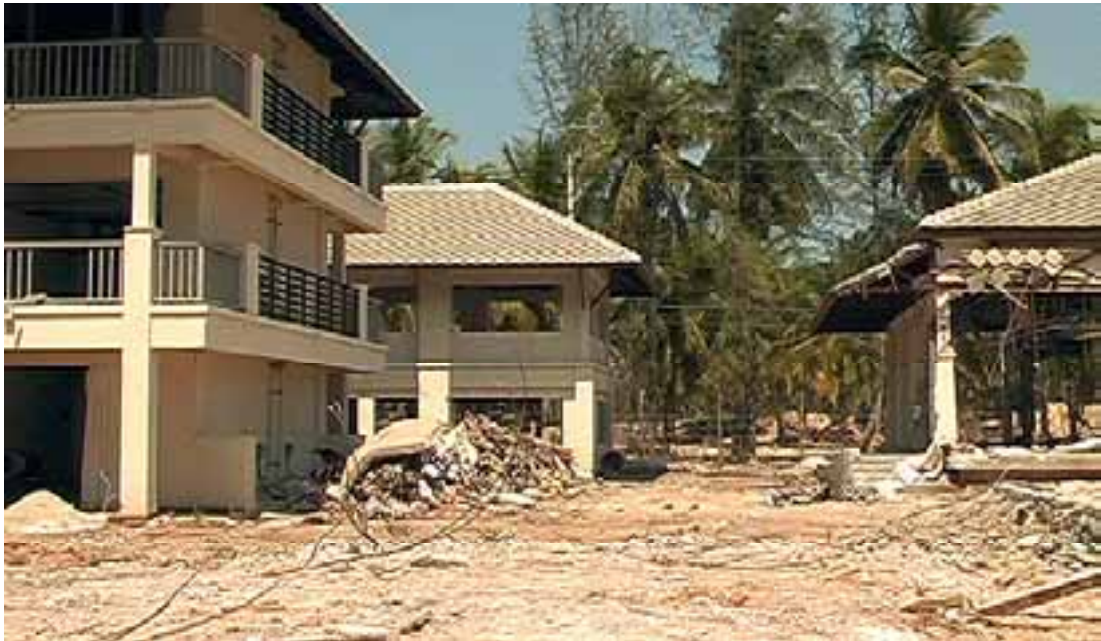
Figure 17. Sturdy buildings survived, especially if they had light walls and windows that were not load bearing and which could collapse due to water pressure. The top floors of three storey houses remained totally intact.
