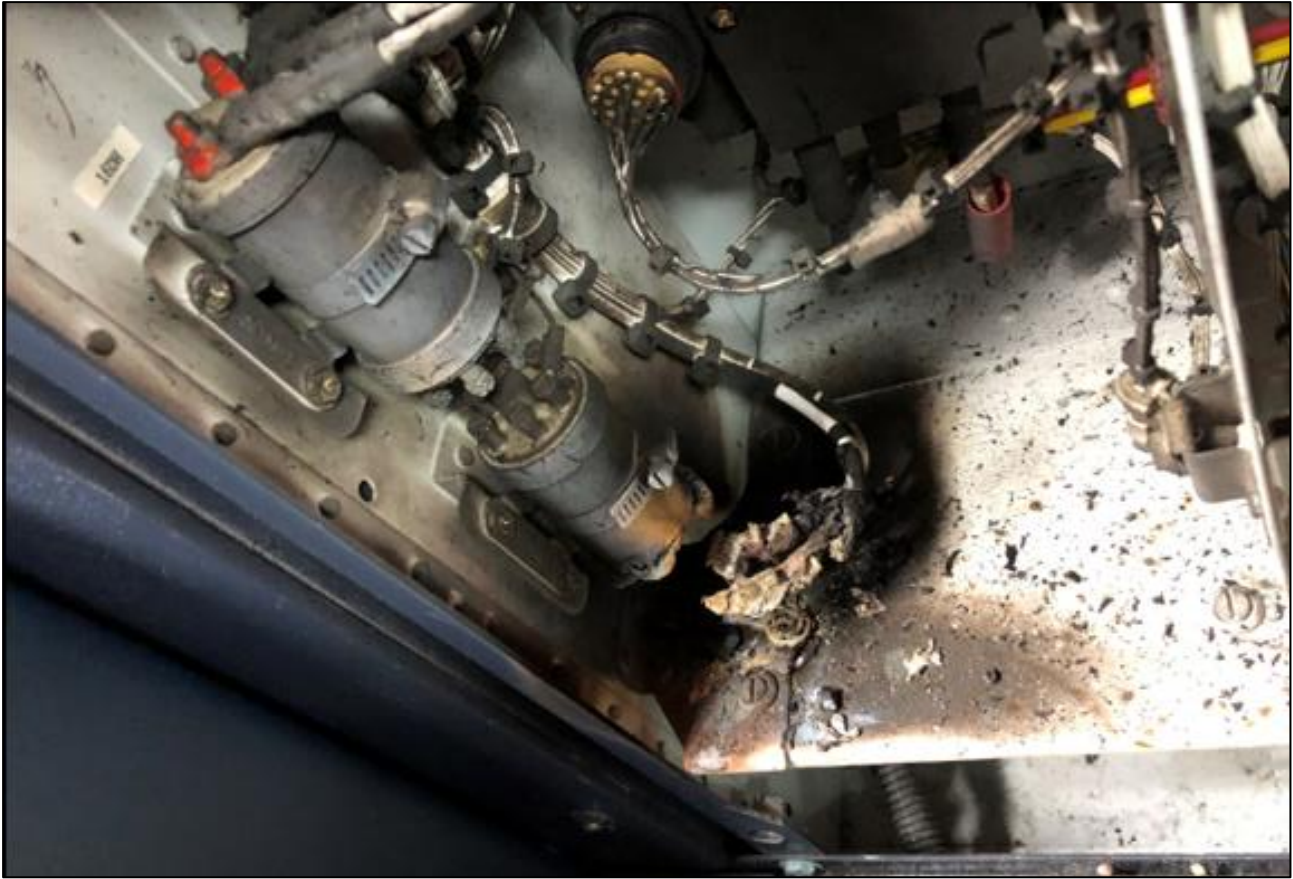
Figure 4. The burnt anti-icing system relay, the photo was taken before repairs. (Photo: Norra)
