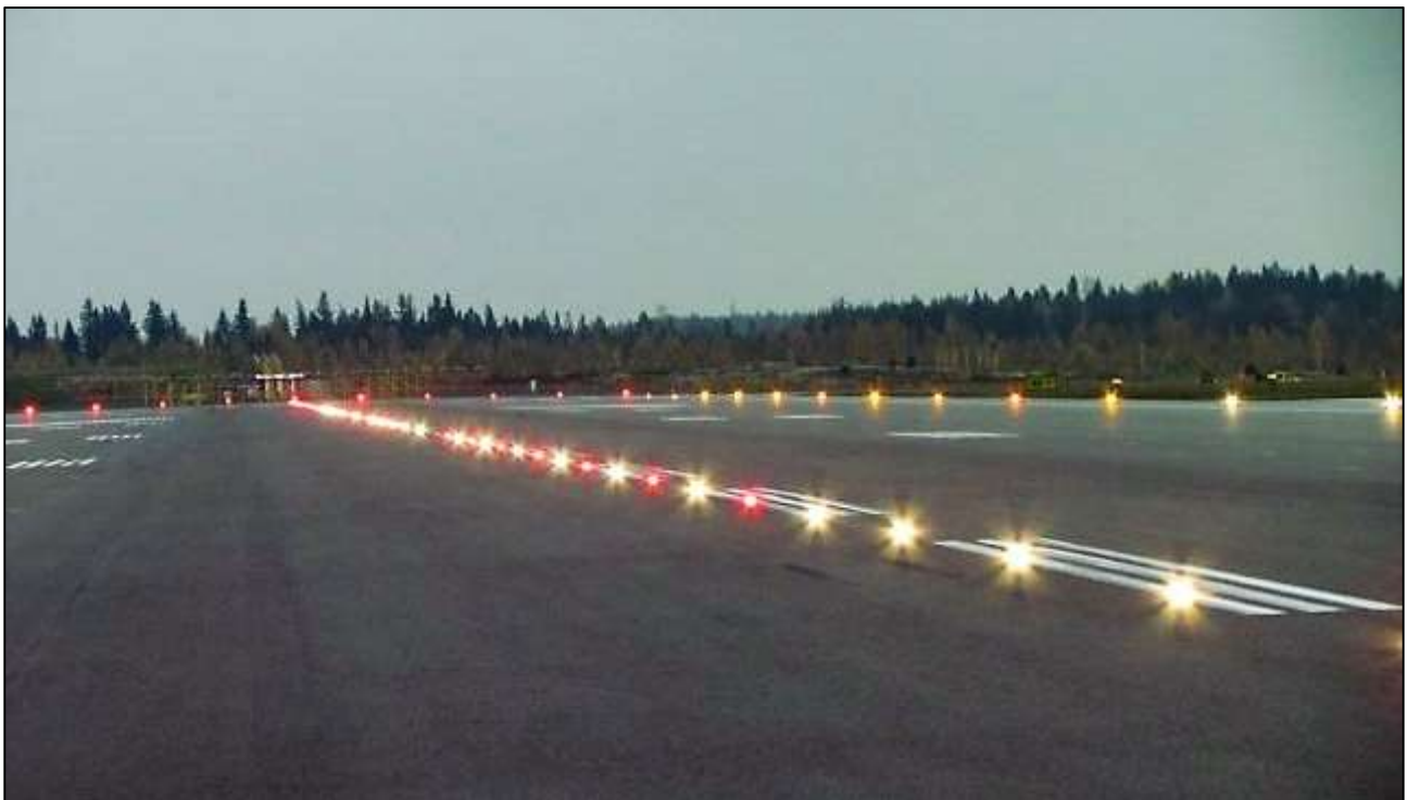
Picture 3. The final 900 m portion of the runway is indicated by alternating red and white centerline lights. (Photo: SIAF)
