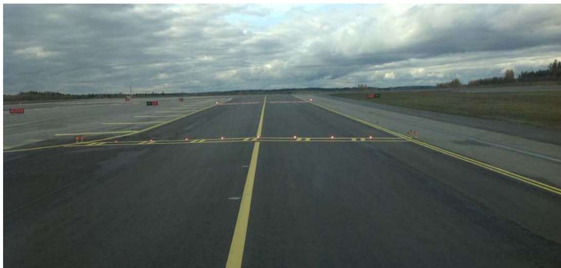
Figure 2. The stop bar on taxiway WD.
