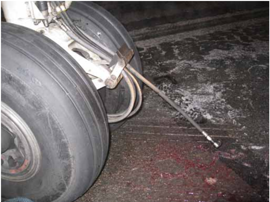
Figure 2. The brake line broken at the swivel as well as a pool of hydraulic fluid on the ground
