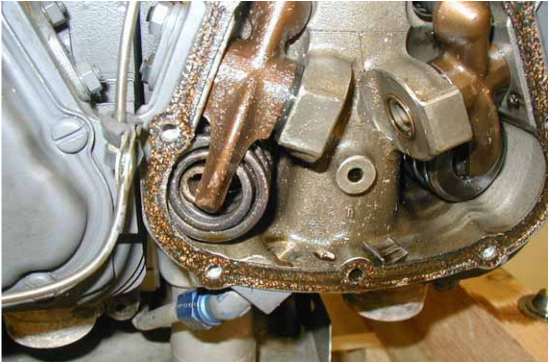
Figure 4. The intake valve of cylinder number 1 had moved into the cylinder.
